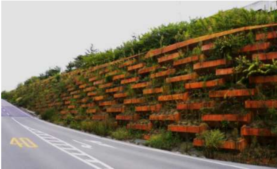
Evergreen GEO: Motorway Bridge Abutment, wall built in Japan along Highway Tokyo - Osaka
